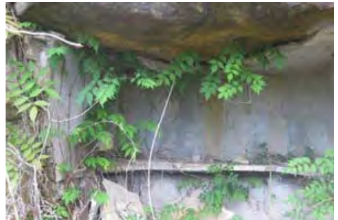
Photo 17: 'Cool room' formed of steel and concrete lining.
