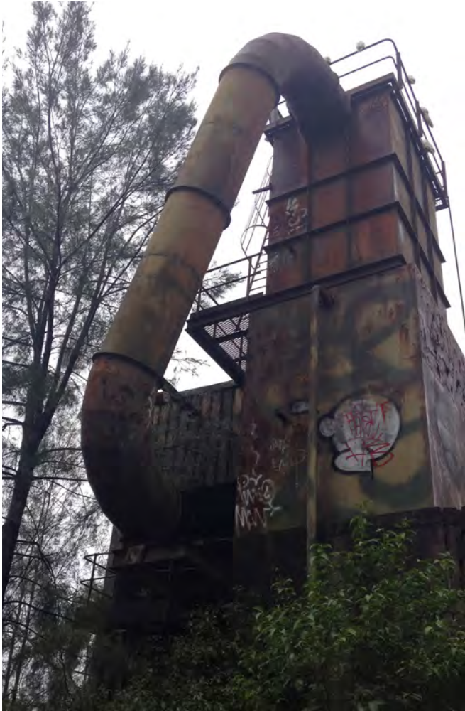
Photos 27: Old crusher plant building
