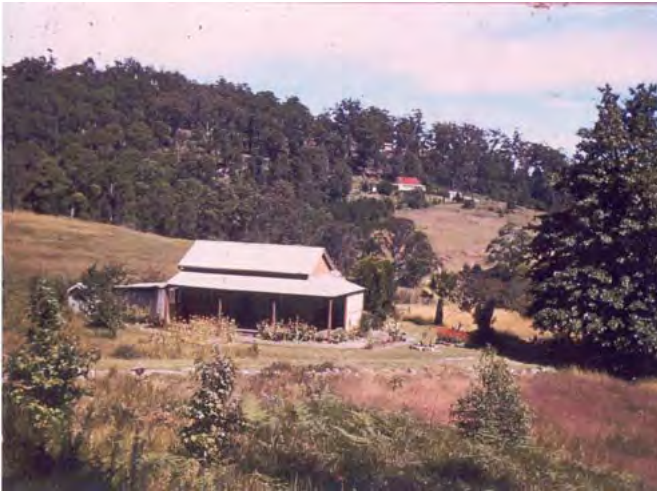
Photo 9: Two of the former Higgins family homes are seen here in OMV and in the adjoining Hornsby Quarry lands c. 1959, before being demolished by Farley & Lewers to make room for the expansion of quarrying operations.
