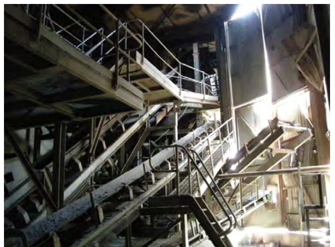
Photos 30: Old crusher plant machinery
