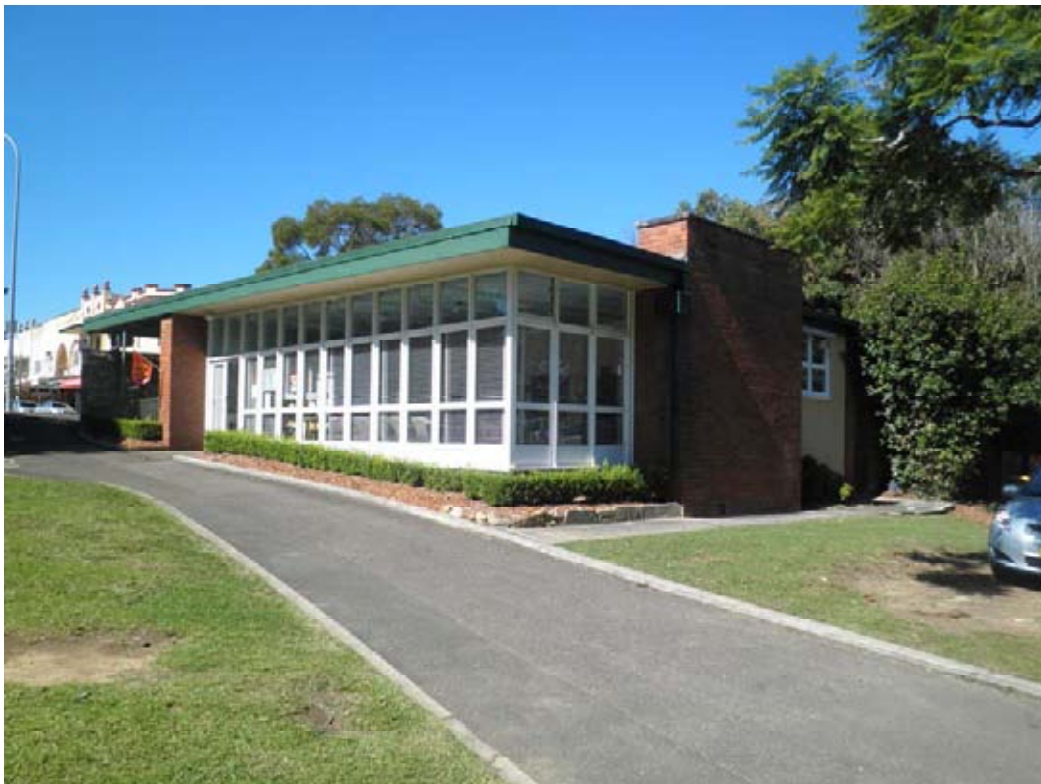
Hornsby & District CWA Women's Tea Rooms & Rest Centre front (north) façade
