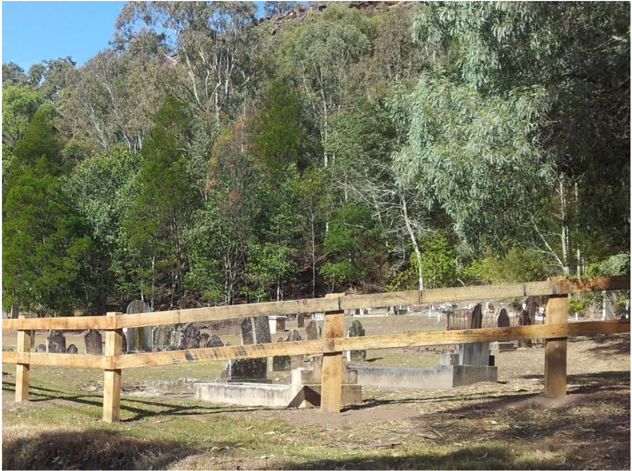
Wisemans Ferry Cemetery fence and asset protection works
