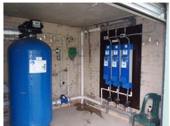
Photo 29: Epping Oval filtration and UV system
