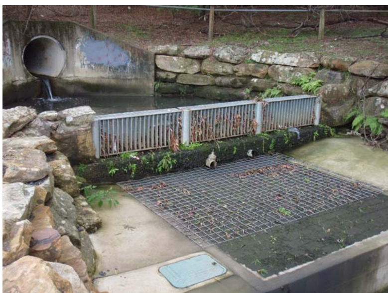
Photo 27: Stormwater harvesting collection point near Berowra Oval. After passing through a trashrack the stormwater is filtered through permeable pavers and collected in an underground concrete tank from which it is pumped on demand to the UV treatment system at the nearby oval.
