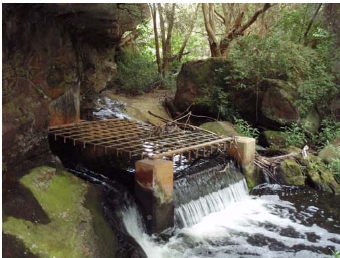
Photo 15: discharge point for treated sewage into Calna Creek below Hornsby Heights STP
