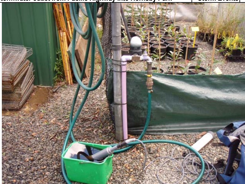
Photo 6: Site 98 Council’s Nursery at Pennant Hills. Stormwater is captured, treated and stored for use on site for nursery irrigation and toilet flushing. The mauve pipes differentiate the stormwater and potable townwater supply.
