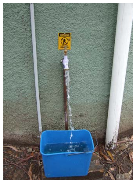
Photo 28: Site 132. Foxglove Oval at Mount Colah. Sampling tap on the header tank where irrigation water is stored.
