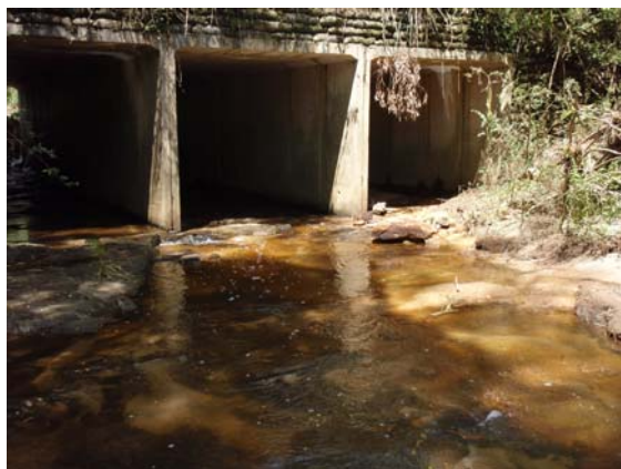
Photo 20: Site 42 Colah Creek under Wylids Rd near Glenorie
