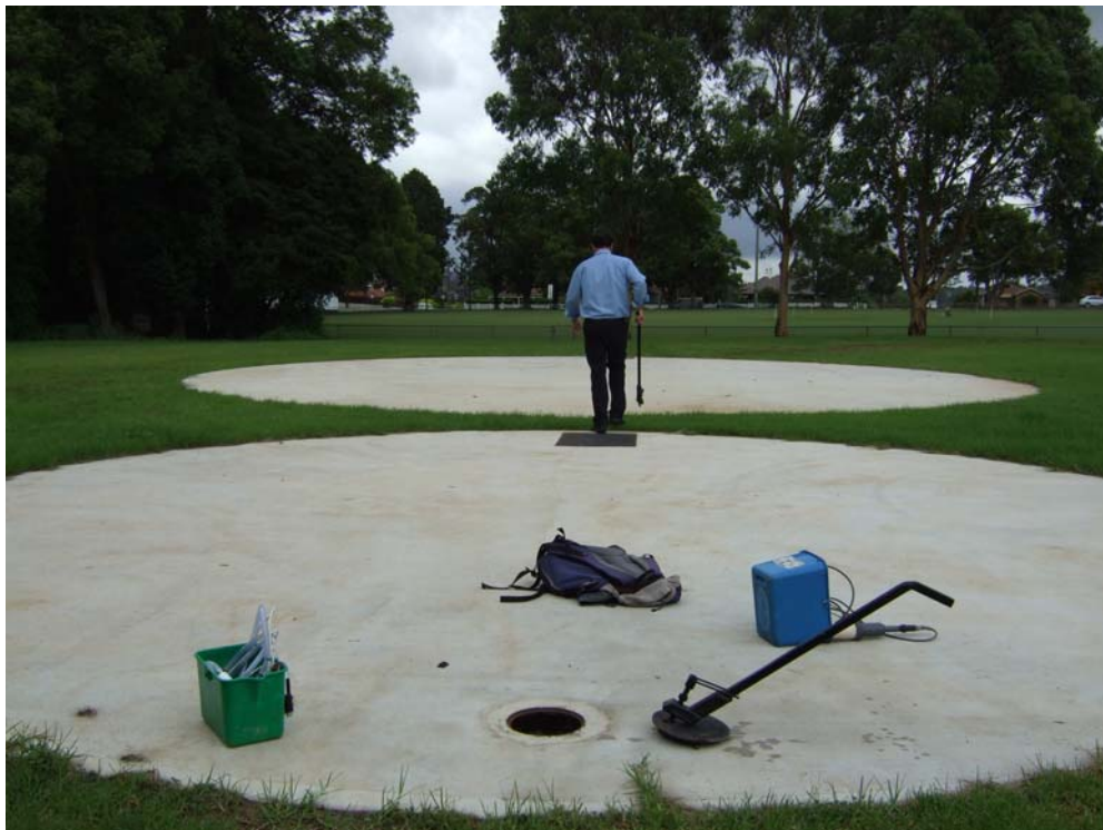
Photo 4: Tanks at Epping Oval for holding stormwater harvested from nearby streets
