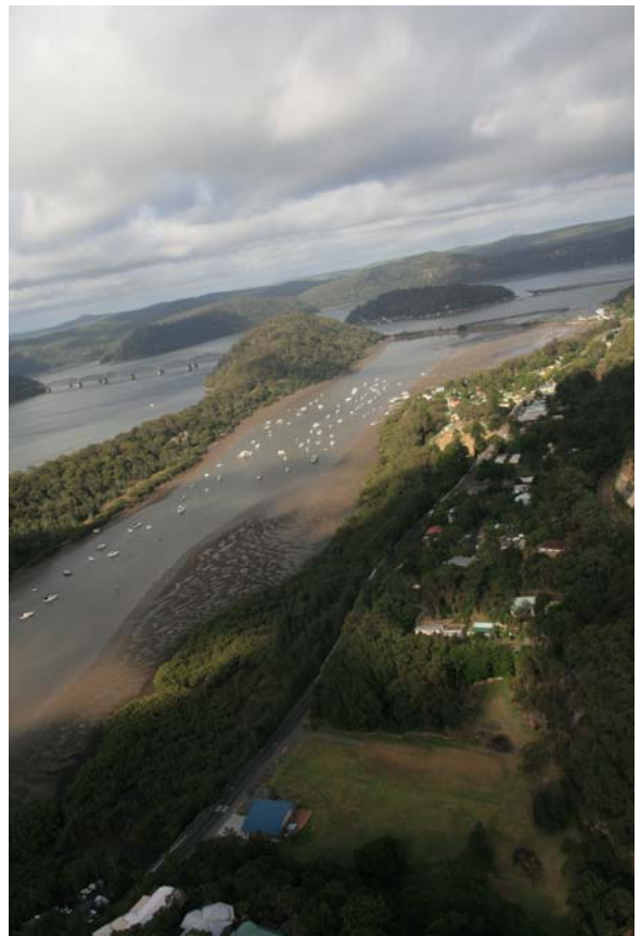
Photo 1: Aerial view of Sandbrook Inlet at Brooklyn with rail bridge over the Hawkesbury River in the background
