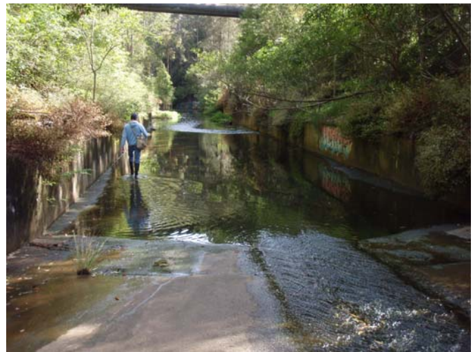
Photo 16: Waitara Creek flowing through a concrete culvert past West Hornsby STP. The discharge point for treated sewage is seen on the right side underneath the overhead sewer main.
