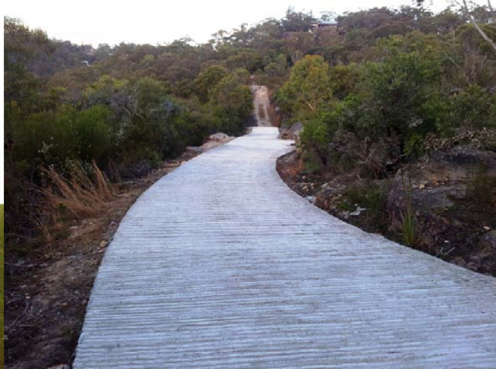
Woodcourt fire trail stage 3 works
