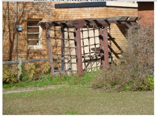
Caption: Relatively rare timber garden arbour in need of repair / restoration. Side fence is original timber-framed type with wire mesh panels. Copyright: GML 2012 Image by: Musecape for GML Image Date: July 2012 Image Number: Image Path: Image File: Thumb Nail Path: Thumb Nail File:
