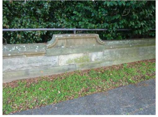
**Caption:** Detail of front fence which previous Heritage Study assumed may have been recycled from a historic building. Fact that moulding on higher centre section does not align with that on fence capping supports this theory.
