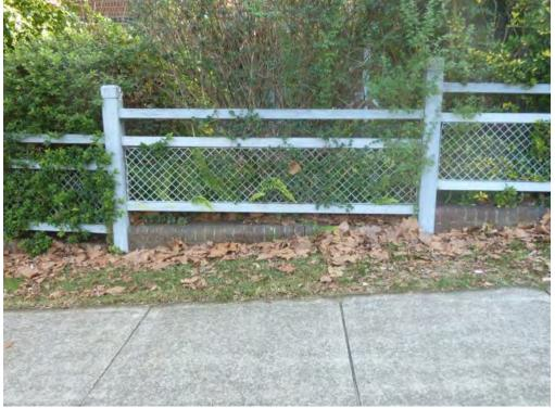
Caption: Fine timber post and wire mesh panel front fence on bullnose brick dwarf wall. Copyright: Chris Betteridge, Musecape for GML, 2012 Image by: Chris Betteridge, Musecape for GML, 2012 Image Date: April 2012 Image Number: Image Path: Image File: Thumb Nail Path: Thumb Nail File:
