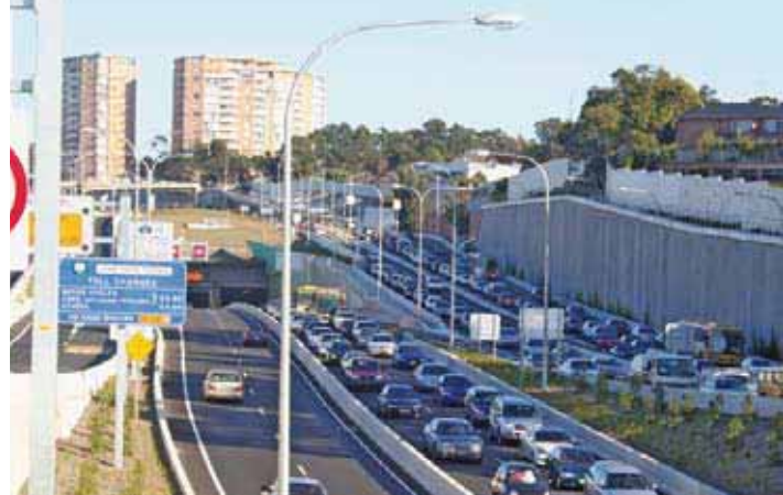
East bound traffic coming out of the Lane Cove Tunnel
