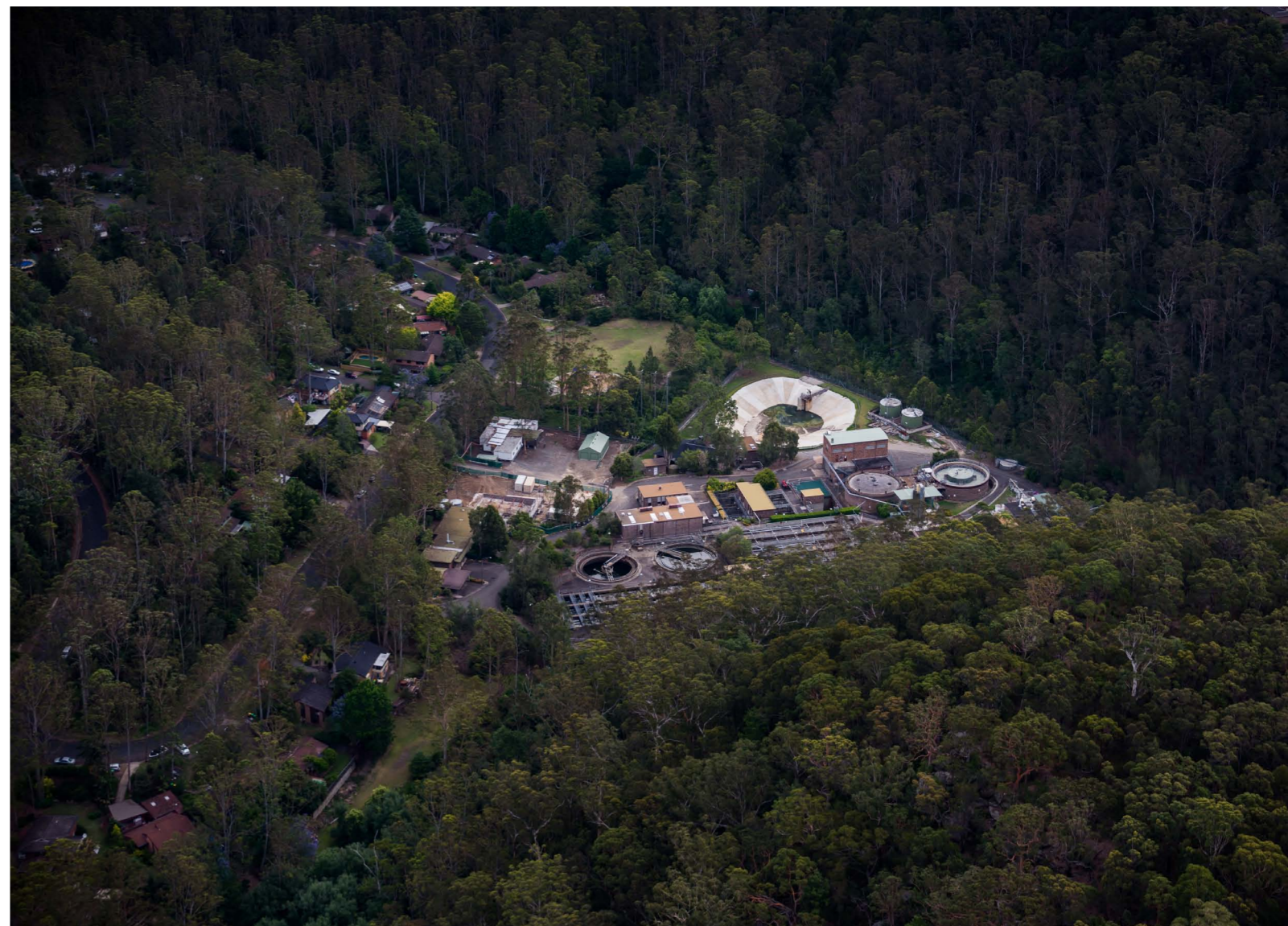
Figure 7.8: Aerial view of West Hornsby Sewage Treatment Plant
