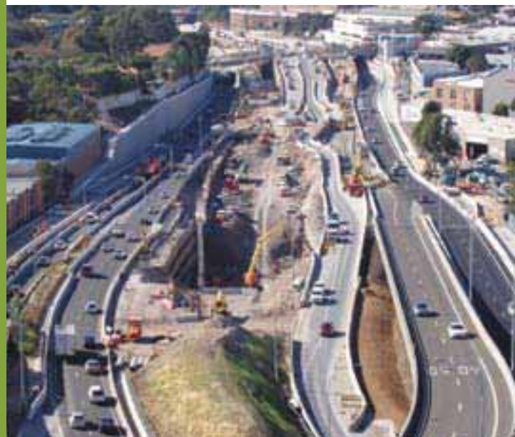
The Lane Cove Tunnel under construction
