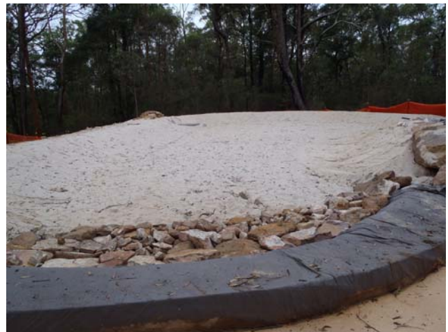
Plates 2-6: Dawson Avenue, Thornleigh - Bioretention Basin and Stormwater Harvesting System Constructed in January 2013.
