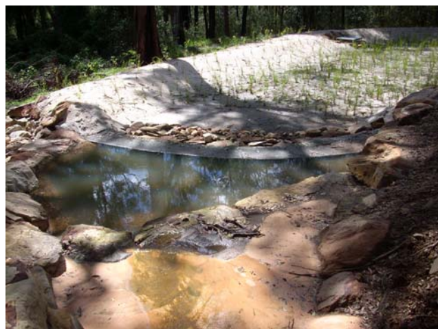
Plates 2-6: Dawson Avenue, Thornleigh - Bioretention Basin and Stormwater Harvesting System Constructed in January 2013.
