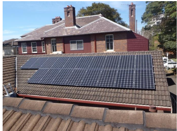
Willow Park photo voltaic cells
