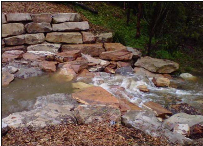
Plate 13 – Valley Road, Hornsby – Bank and spillway repair
