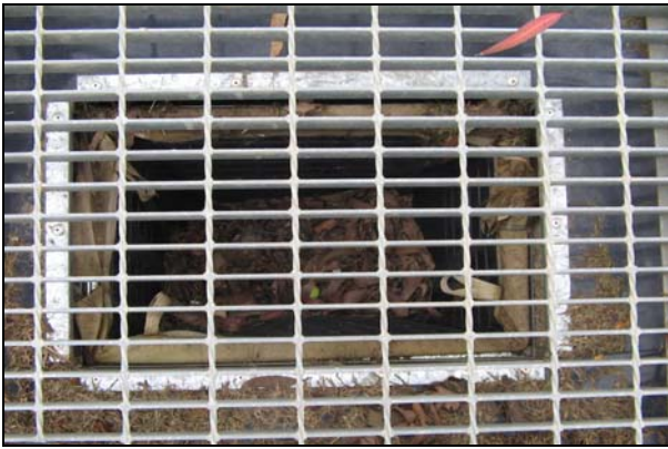
Plates 7 & 8 – Newly installed Pit Inserts, Blaxland Road (Somerville Park), Eastwood.
