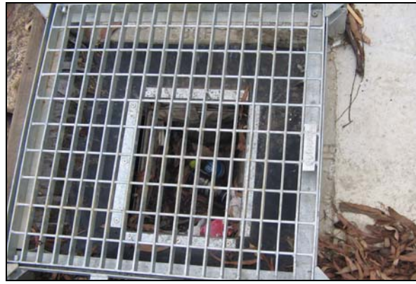
Plates 7 & 8 – Newly installed Pit Inserts, Blaxland Road (Somerville Park), Eastwood.
