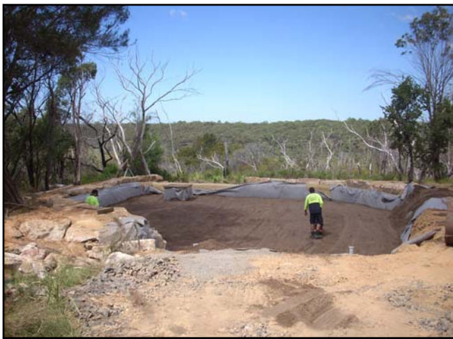
Plates 2, 3, 4 & 5 – Church Street, Mount Kuringai - Bioretention basin during construction and after planting.
