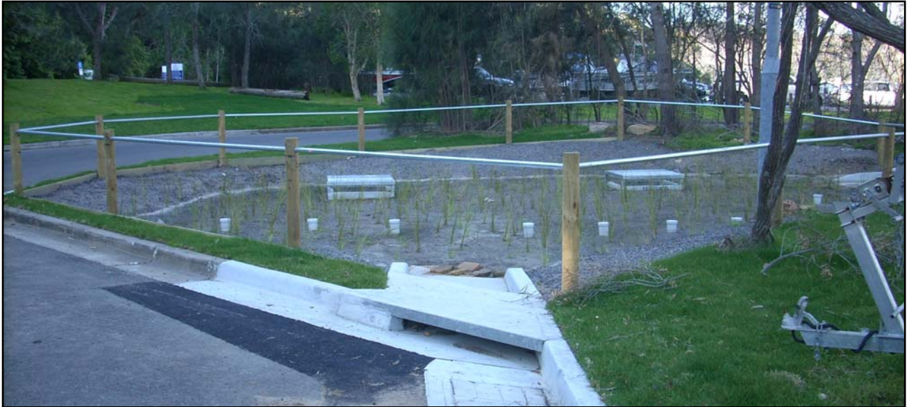
Plate 6 – Parsley Bay, Brooklyn – Carpark raingarden during construction and after planting
