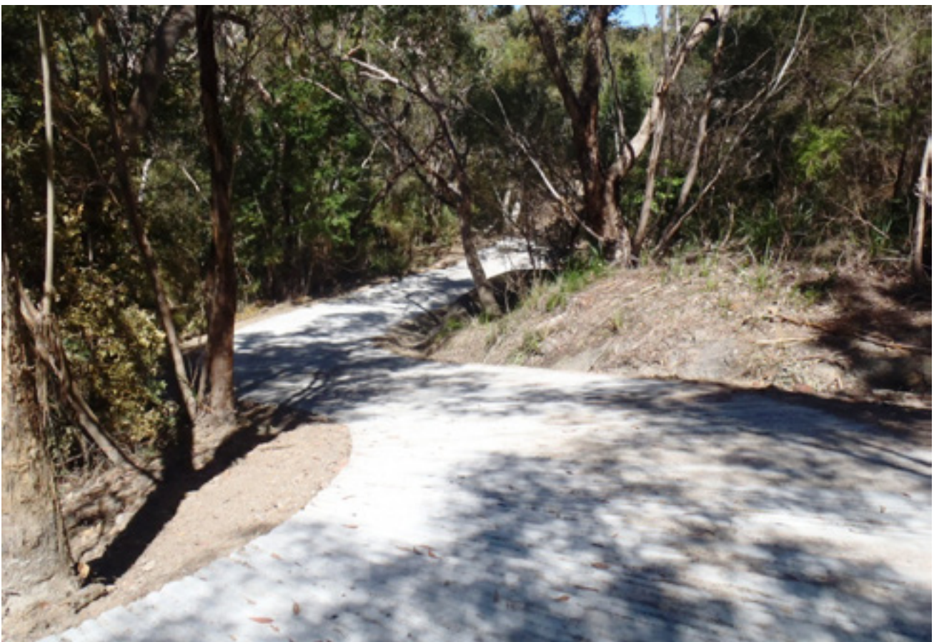
Stage 1 of the Woodcourt Fire Trail upgrade at Berowra completed in 2011-2012 (Photo: Phil Murdoch)
