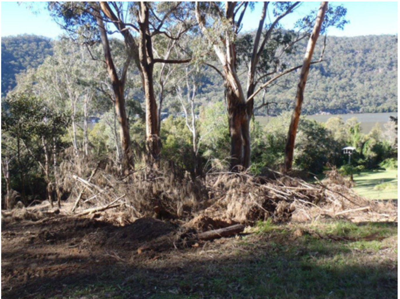
Unapproved vegetation clearing works for Asset Protection Zone not done in accordance with Planning for Bushfire Protection 2006 in Wisemans Ferry area (Photo: Alex Fraser)
