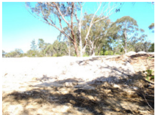
Unapproved landform modification including significant amounts of imported fill (Photo: Alex Fraser)
