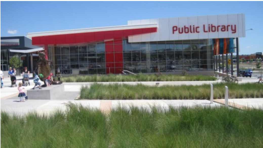
Figure 17: Vinegar Hill Library (top) and Gungahlin Town Centre Wellbeing Precinct (bottom), examples of larger, clustered facilities in town centre locations
