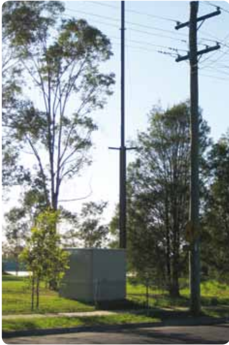
A typical air release facility
