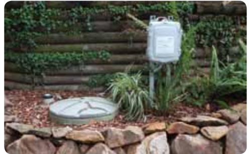
Examples of installed pressure sewerage equipment
