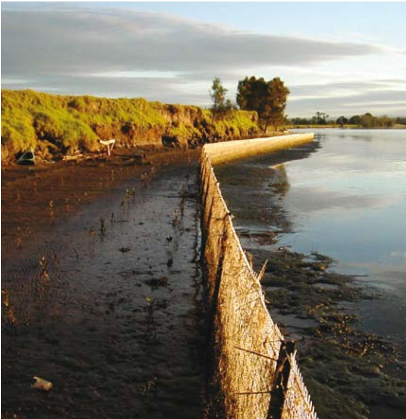
Figure 18: Mangrove seedlings planted in front of an eroding bank along the Shoalhaven River, with the use of temporary mesh fencing as a wave barrier and to protect establishing mangroves from debris. Photo—Allan Lugg, Department of Primary Industries.
