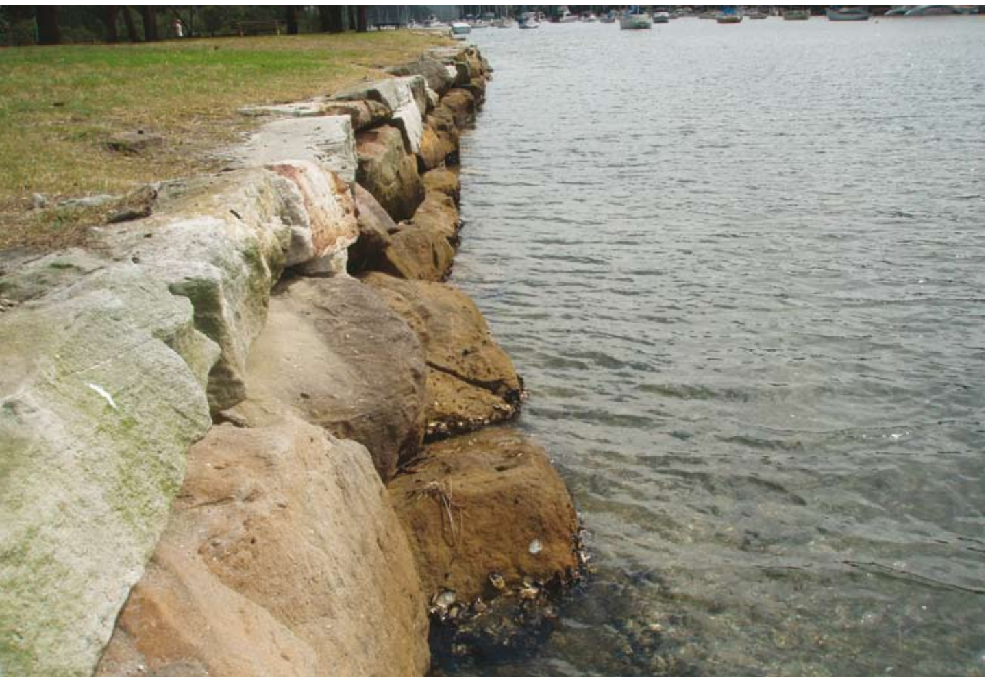
Figure 22: Example of a seawall made from boulders of various size and shape placed together without cement in McCarrs Creek, Pittwater.
