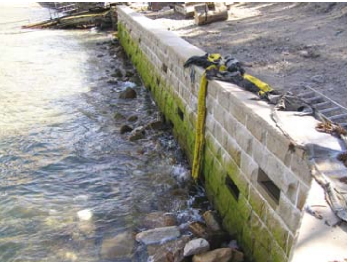
Figure 24: A seawall at McMahons Point, Sydney Harbour, purposely designed to include pools in the structure for habitat, and boulders at the toe for additional habitat.
