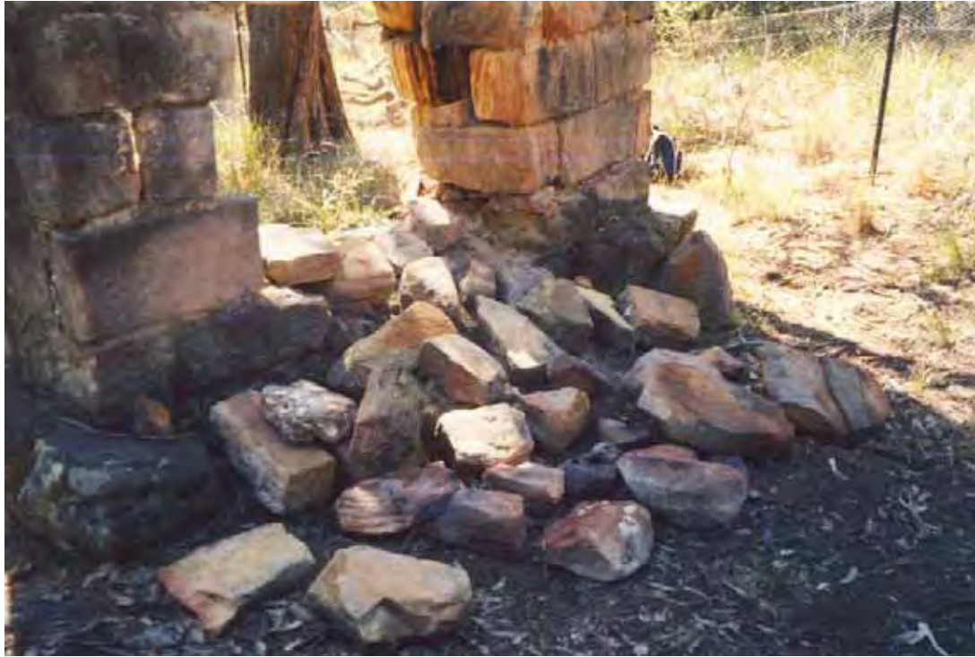
Photo 6. Adjacent stones to chimney
