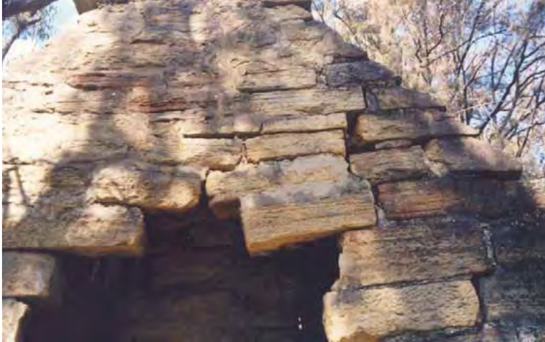
Photo 2. Detail of collapsing section of chimney
