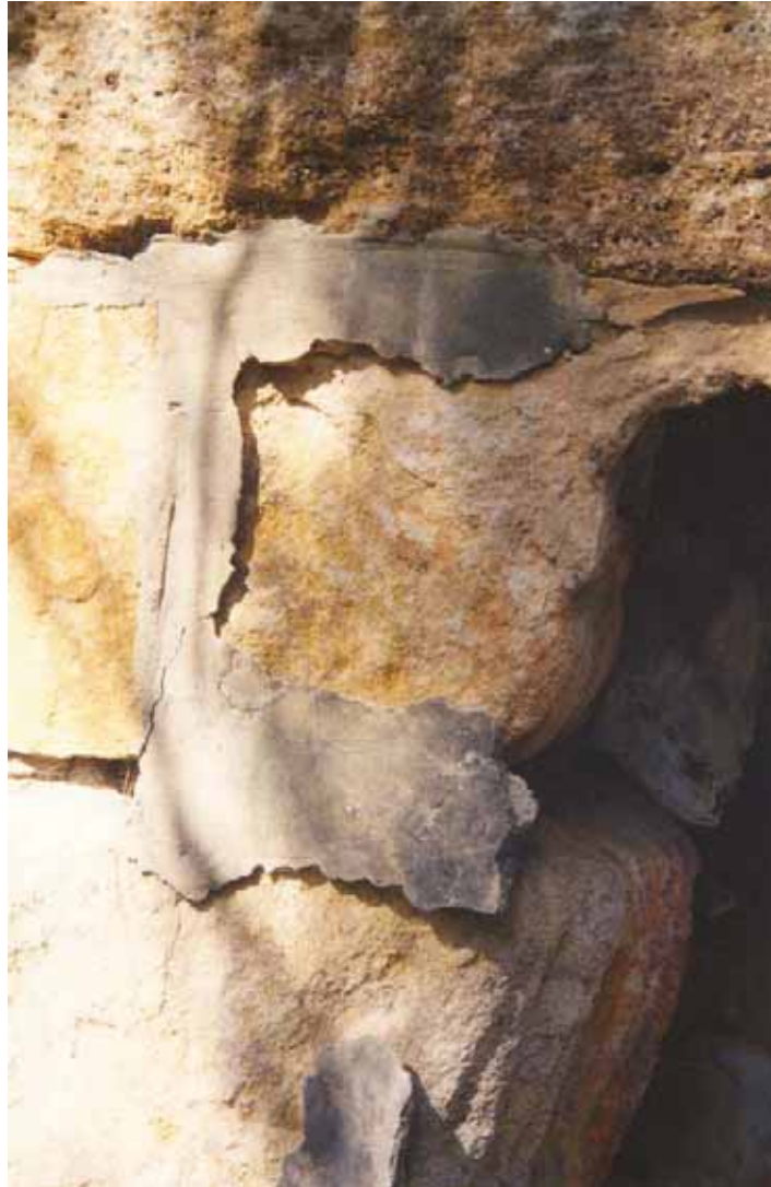
Photo 3. Inappropriate repointing with adjacent stone exfoliation
