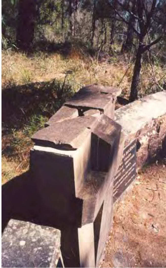
Photo 7. Damage to Memorial Lookout capping
