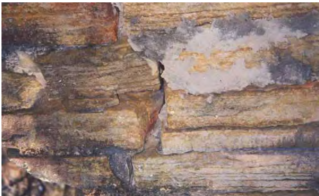
Photo 4. Inappropriate repointing
