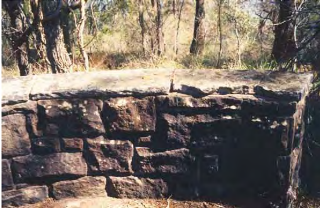
Photo 8. Damage to end coping stones on Memorial Lookout
