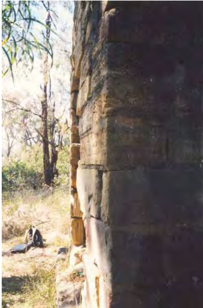
Photo 5. Belying out of north face of chimney
