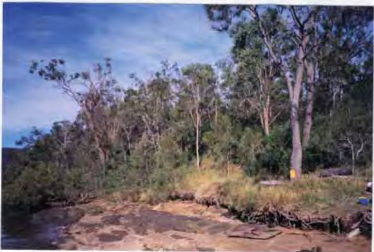
Figure 2 Bar Island - north eastern shore at site of derelict jetty. Embankment undercut by wave action.
