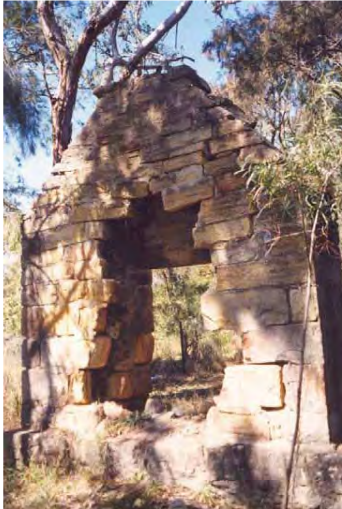
Photo 1. Chimney showing loss of stone
