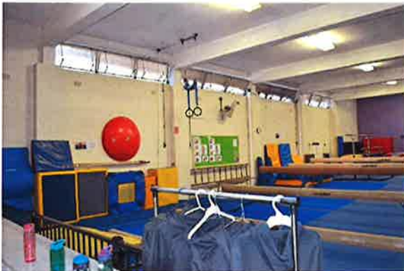
18. Lower Hall- wall adjoining Ashley Lane.
